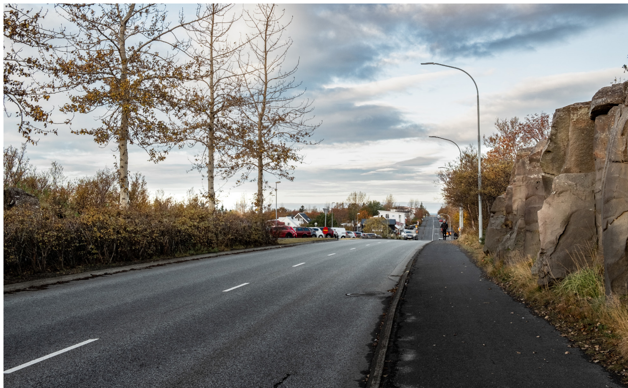
Fig. 22 - Existing conditions on section 180
